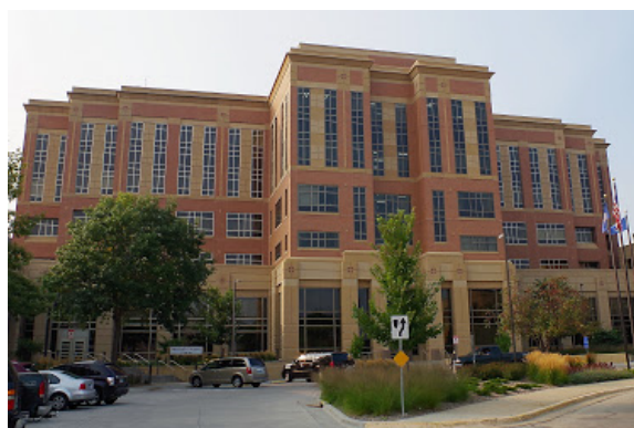
Olmsted County Court House
